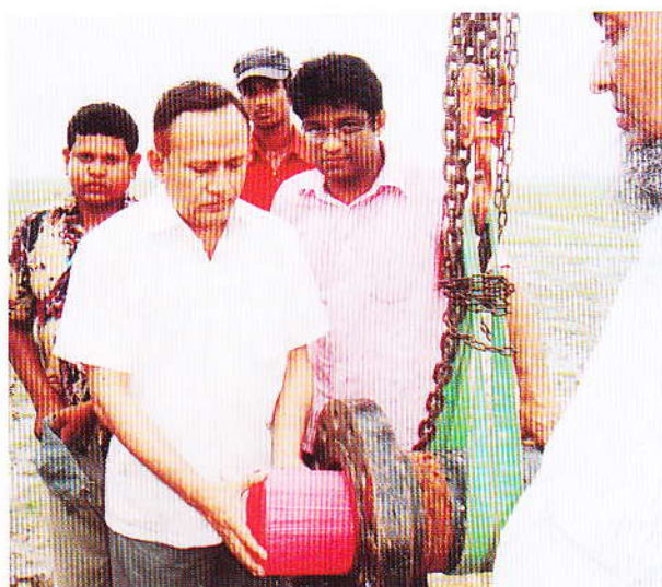
A view of the Pigging Works at Nobiganj area under Nobiganj Gas Supply and Distribution Project.
